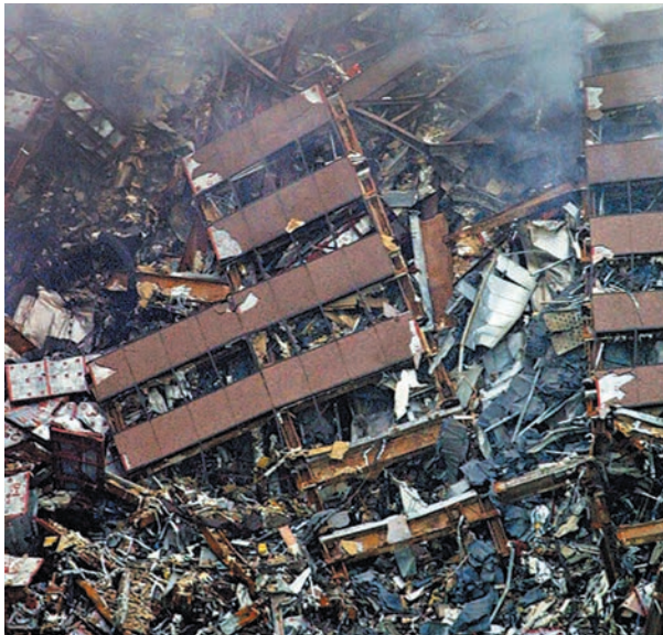
The wreckage of Building 7 two days after 9/11.
