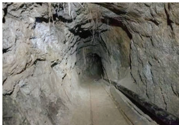
This Border Patrol photo shows the unfinished tunnel that stretches from Jacume, Mexico, to Jacumba, San Diego County, Calif.
